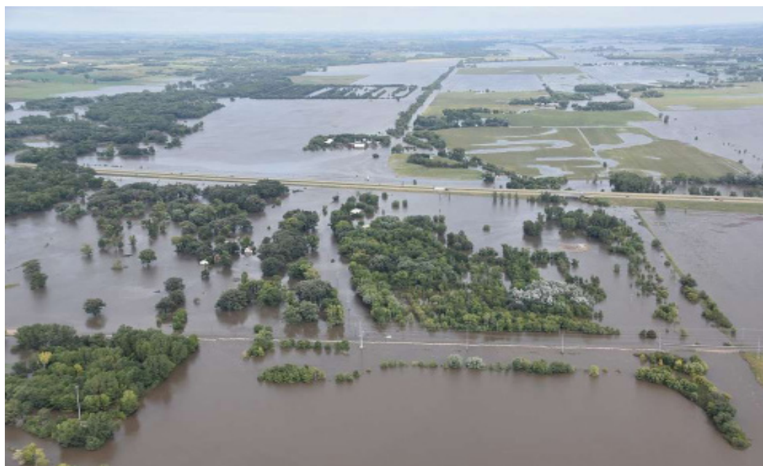
Big Sioux River Flooding at Interstate 90 in South Da-
